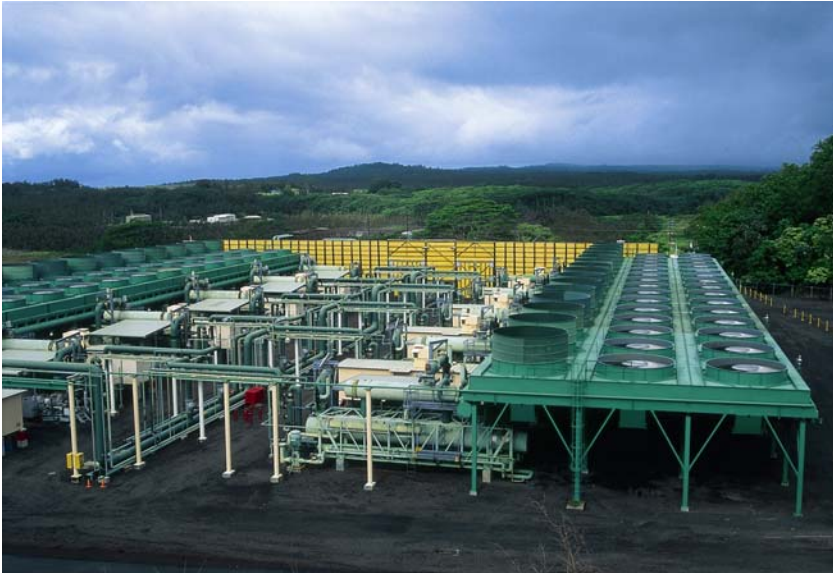
Figure 20: Puna Flash/Binary Geothermal Plant
